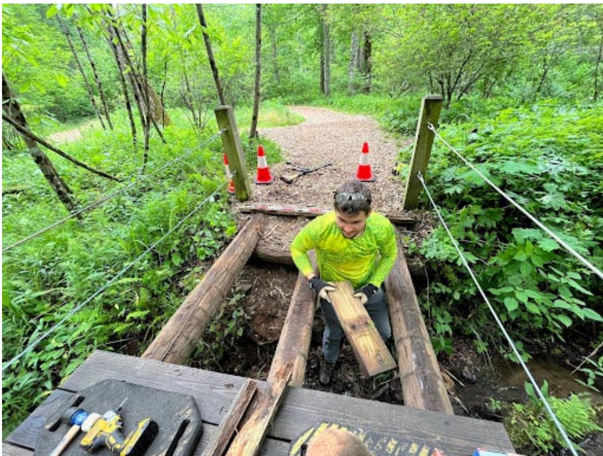
Figure 5. Infrastructure updates in the Native Azalea Collection have improved visitor experience and safety. Here, North Carolina Arboretum staff member Luke Sheaffer assists with redecking one of the Collection's bridges. Photo by Carson Ellis.
